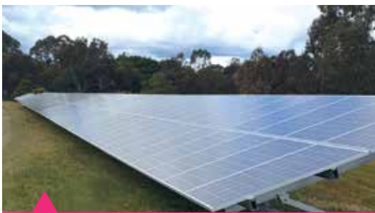
THE INSTALL: 99KW GROUND MOUNT SOLAR SYSTEM
